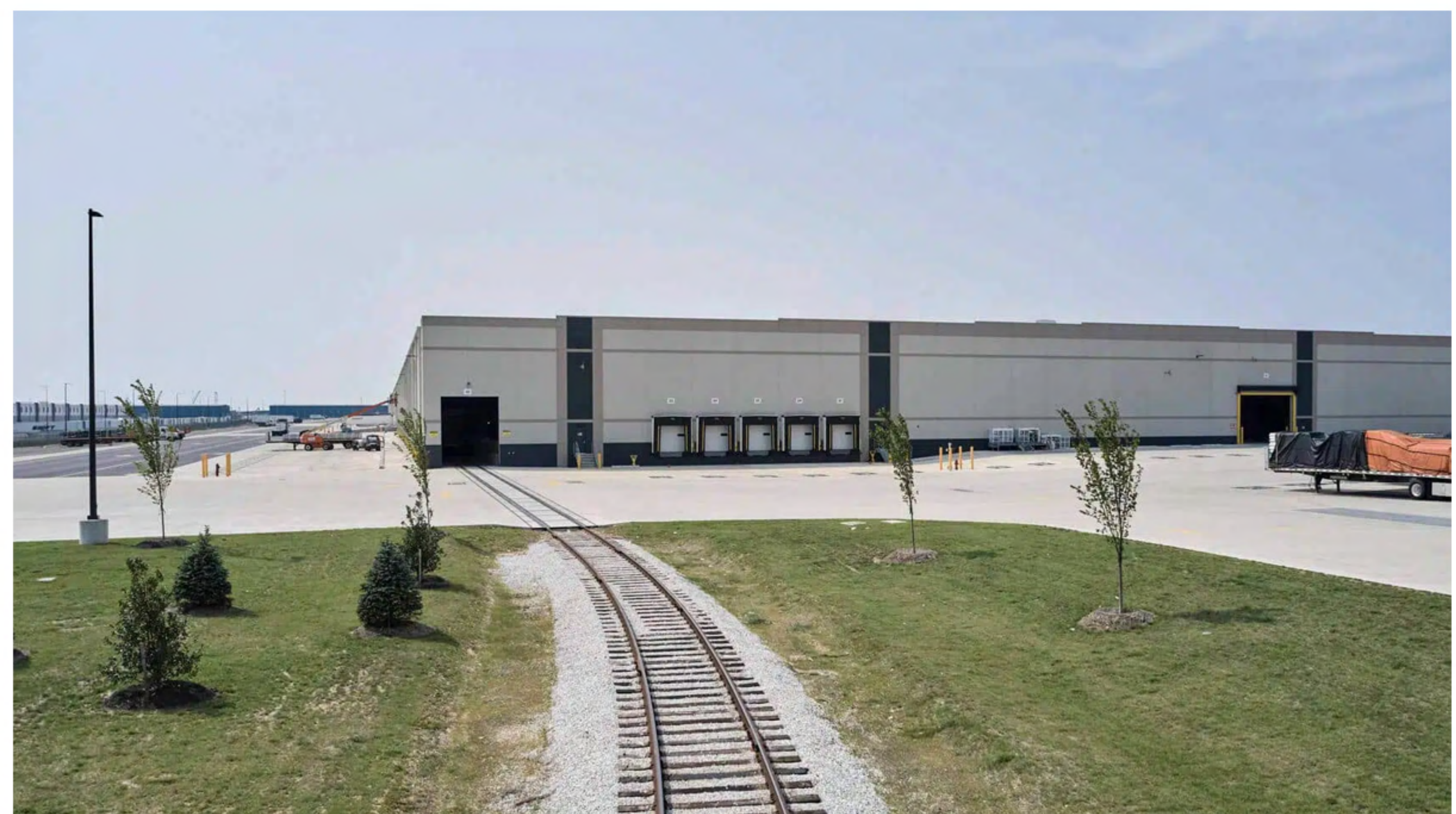
Home Depot Rail-Served Warehouse
